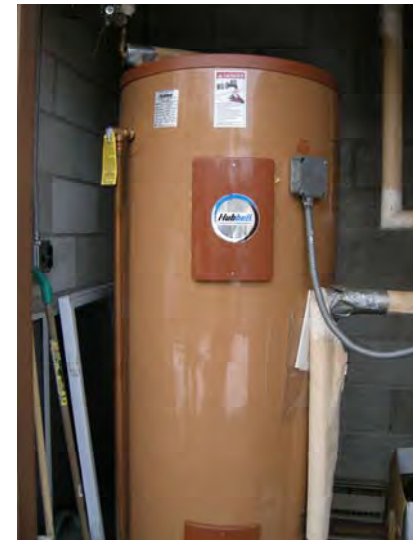
Typical electric water heater
