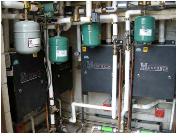
Gas-fired high efficiency heating boilers
