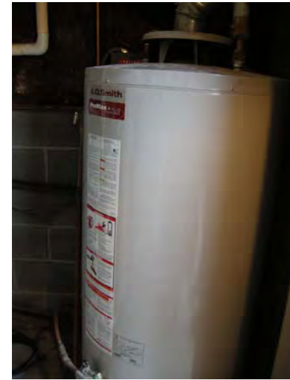
Gas-fired hot water heater
